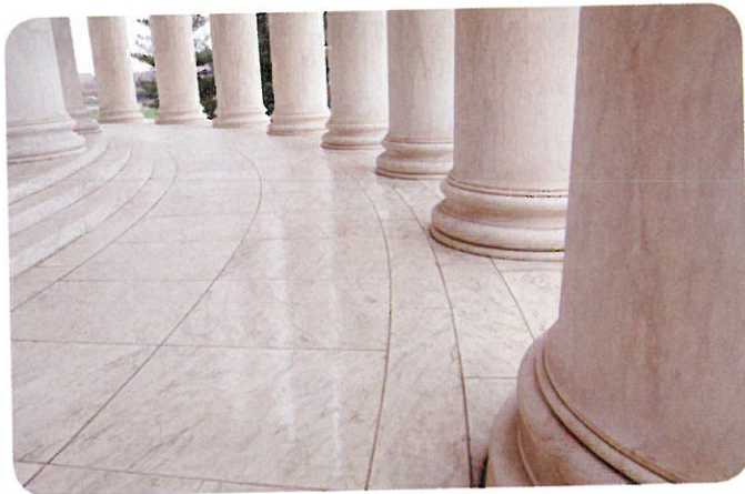
■ Figure 6.22 Marble and slate are metamorphic rocks that have been used in construction for centuries.
